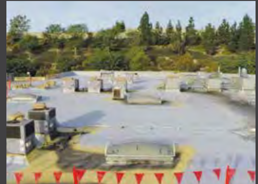
View of partially completed ccSPF installation
